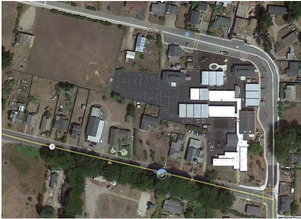
POINT ARENA ELEMENTARY SCHOOL
