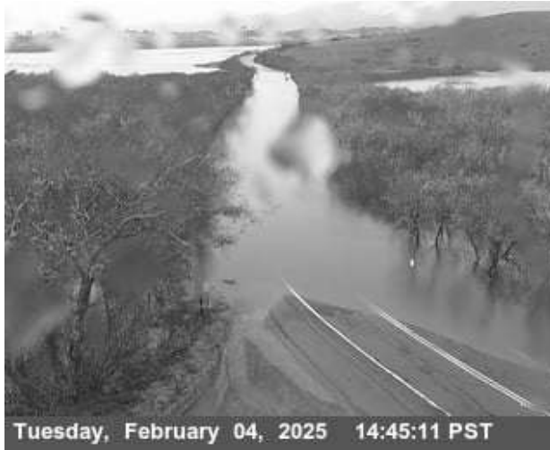
State Route 1 flooded by the Garcia River this afternoon. [Image from Caltrans QuickMap]
