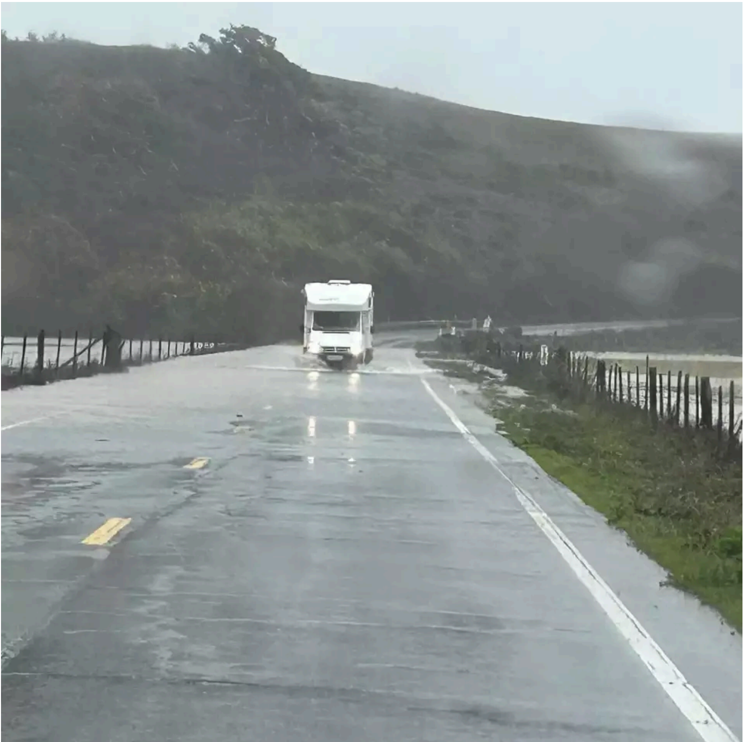
A vehicle crossing the floodwaters of the Garcia River that have closed Highway 1 in Mendocino County, on Nov. 21, 2024. Photograph from Caltrans
